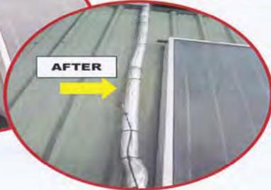
**Don't** lose hot water temperature evaporation from broken or deteriorating hot water insulation covers.
