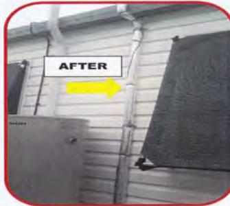
An explanation for the photos of the pipes on your hot water systems. I was contacted by Bill Anderson who noticed a large amount of water around the hot water tank and contacted this plumber. He came out and inspected it and the answer to the problem was the system needed new insulation around the pipes. This new covering has three sections to it, giving a much better result. Have a look at your to make sure it is OK. I did have mine checked.
